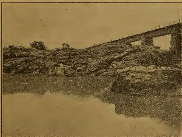
Railway bridge at Zungeru across Kaduna river.
